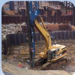
Stone column and wick drain ground improvement for tall walls
