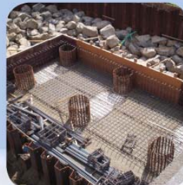
Drilled shaft group with riprap and sheet pile revetment
